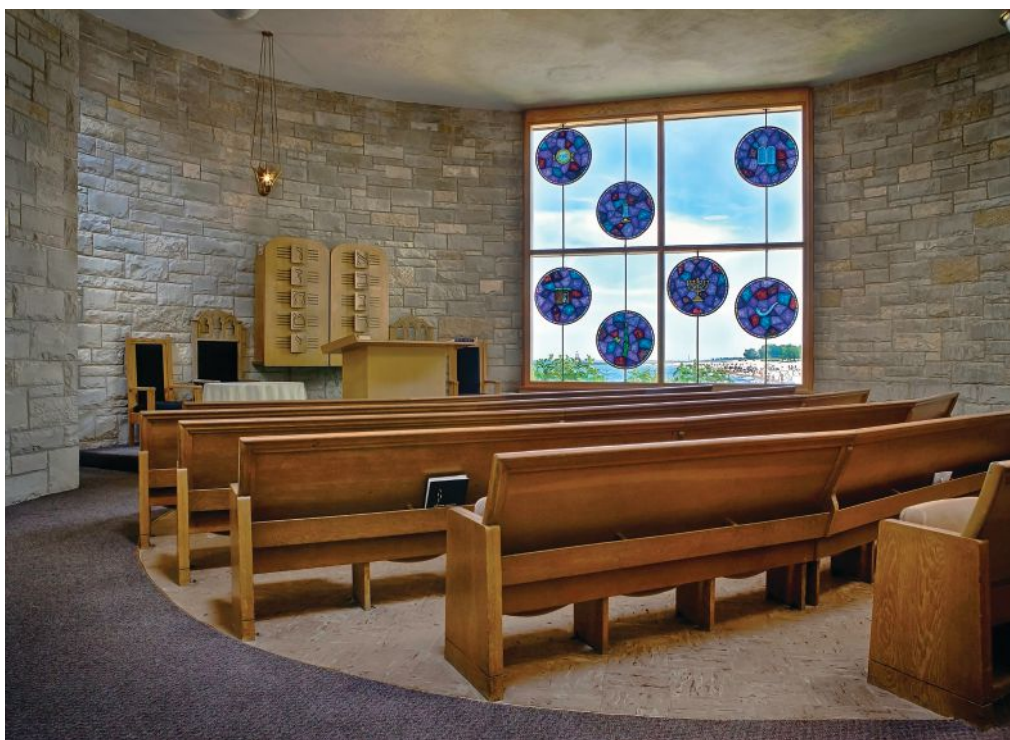
Seen from the neighboring park (top), the chapel's new aperture presents a far warmer image than the solid rock wall had in the past. Cutting open the stone wall (bottom) to create a window and showcase the donated stained glass panels gave the chapel a brighter aspect.
